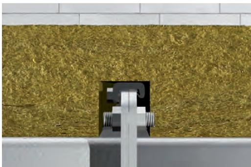
At duct flanges, the slabs need to be cut to fit. The same principle applies for slab joints as well as for slab passages (see picture opposite).
